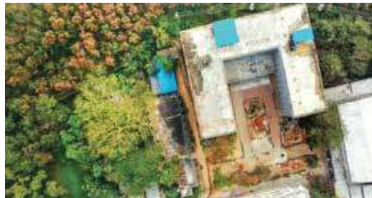
Department of Urban and Regional Planning Building
